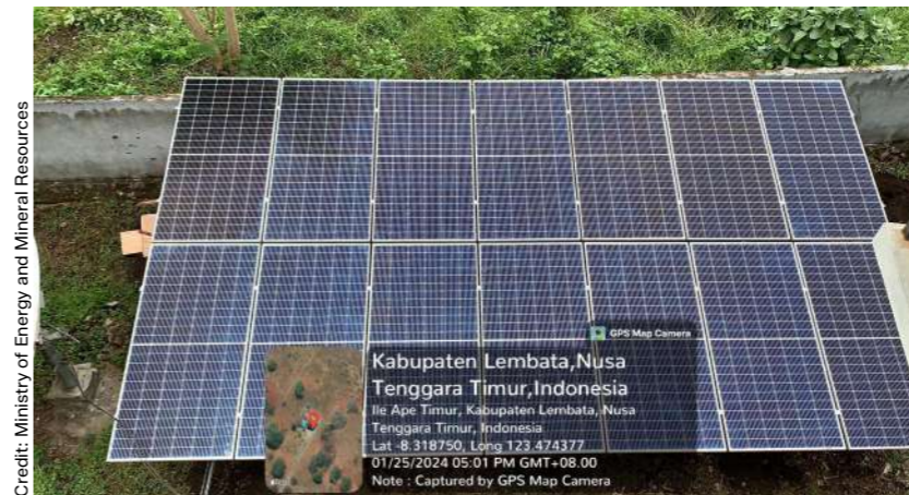
6 kWp solar PV installation at Volcano Observation Post Lewotobi, East Nusa Tenggara.
