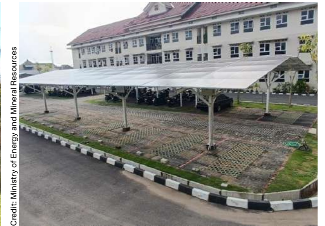
100 kWp rooftop solar PV installation at Yogyakarta Presidential Palace.
